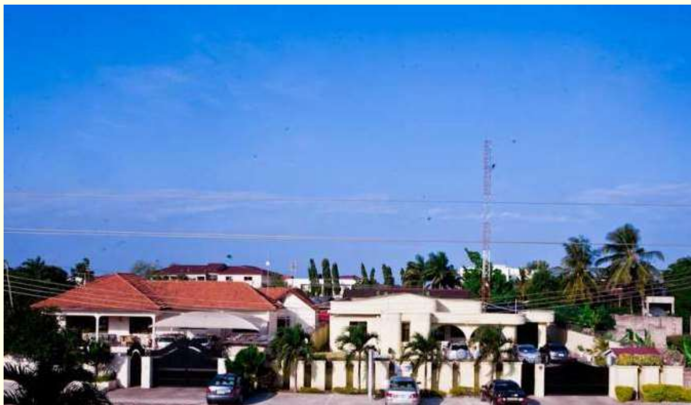
Newly rented building for secretariat staff 38 & 40 Mensah Wood Street at East Legon in Accra, close to GHANA LINK.
